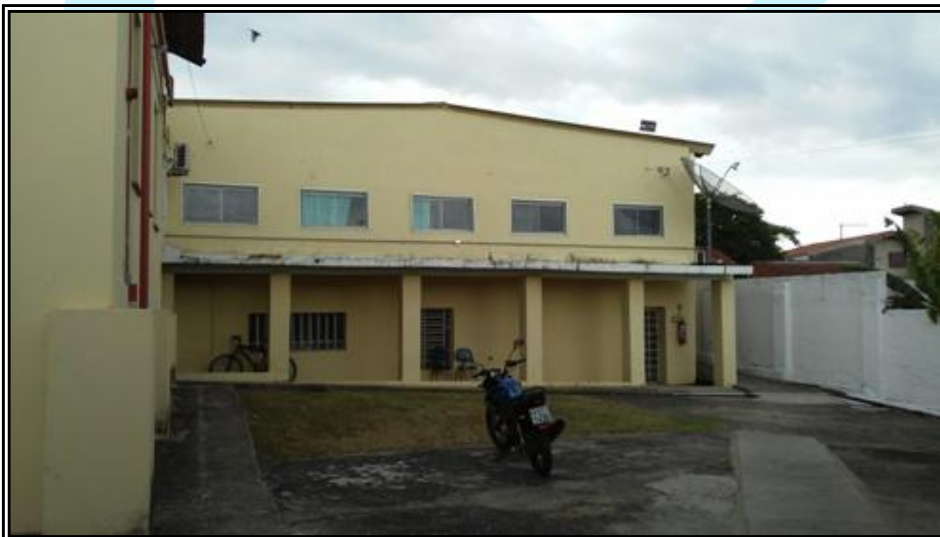
Vista Fundos do Hospital
